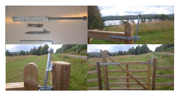
The cane bolt is mounted as shown on the picture. Remember that the higher the position of the gate above the ground, the lower the cane bolt needs to be mounted on the gate in order for the bolt to go far enough into the ground. Open the gate to the desired position and dig down the pipe so that it is positioned level with the ground directly beneath the bolt.
